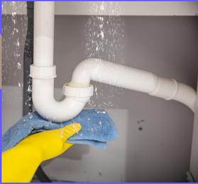
**Note.** Black mould is rarely seen on this type of dampness as the area is usually too wet and the chemicals in a waste waterleak will prevent mould growth.
