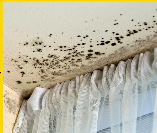
Damp can cause mould on walls and furniture and make window frames rot. Damp housing encourages the growth of mould and mites, as mites feed on mould and can increase the risk of respiratory illnesses in some people. Some damp is caused by condensation. This leaflet explains how condensation forms and how you can keep it to a minimum to reduce the risk of damp and mould.
