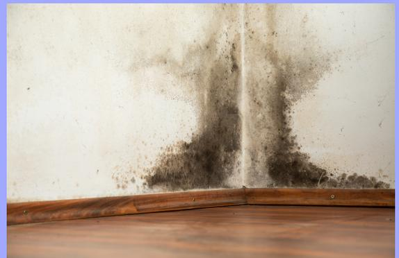
Simply turning up the heating will not sort out the problem. All three factors may need to be looked at to reduce the problem. The first sign of a problem is water vapour condensing on windows and other cold surfaces, which then takes a long time to disappear, allowing surfaces to become damp. The second indication is black mould patches growing on these damp areas.
