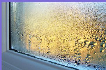
Condensation mainly occurs during the colder months, whether it is rainy or dry outside. It is usually found in the corners of rooms, north facing walls and on or near windows. It is also found in areas of poor air circulation such as behind wardrobes and beds, especially when they are pushed up
