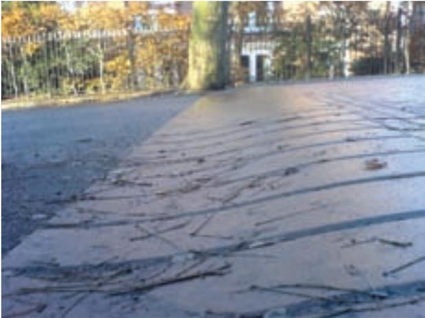
Figure 5.3 Flat-topped hump using pre-formed sinusoidal ramp face units (Tim Pheby)
