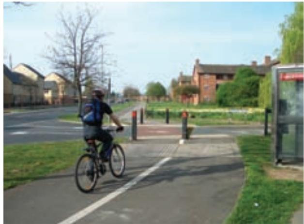
Figure 10.5 Bent-out cycle track crossing (Alex Sully)
