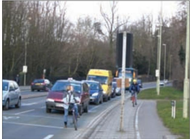
Figure 9.5 Cycle track bypass at a signalised T-junction (Patrick Lingwood)
