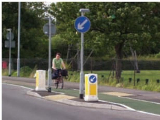
Figure 5.1 Cycle bypass ramped up to footway level (Patrick Lingwood)
