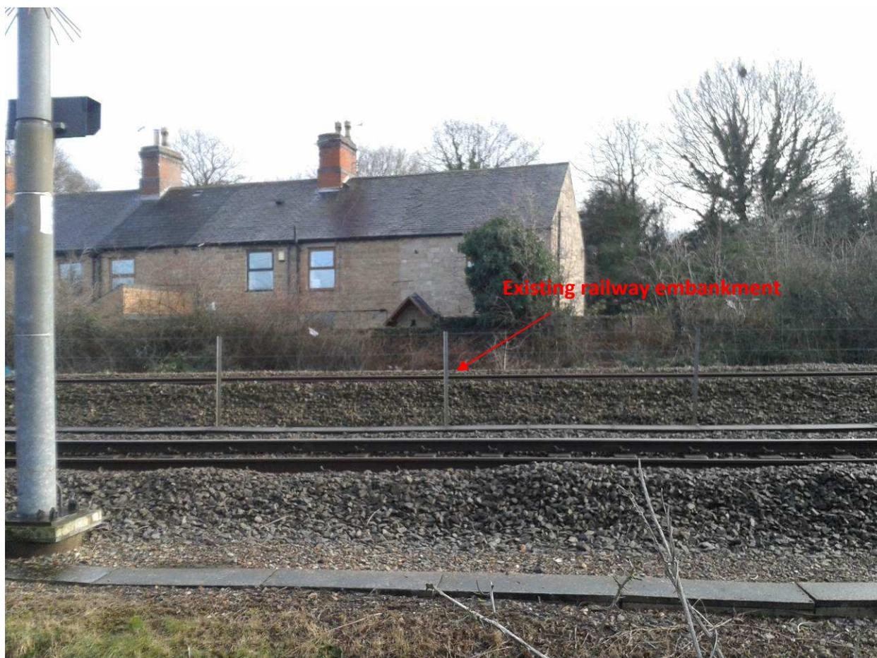
**Figure 4: Existing railway embankment on the west side of Bestwood Road showing the height of the artificial barrier to surface water flow (Facing East)**
