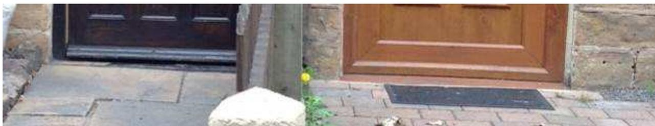
**Figure 5: Low threshold of flooded properties on Bestwood Road allowing water to enter the properties.**
