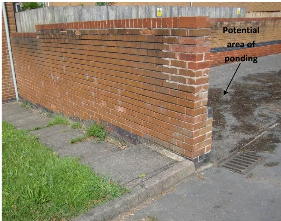
**Figure 5: Brick wall potentially creating a barrier to flow at the north side of Daron Gardens. (N Facing)**
