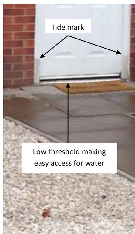
**Figure 6: Example of tide mark and low threshold on Bakewell Drive.**
